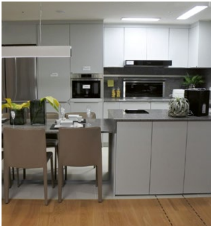
South Korea, Seoul Gaepo Raemian Forest Number of kitchens: 164 Installation: 2020
